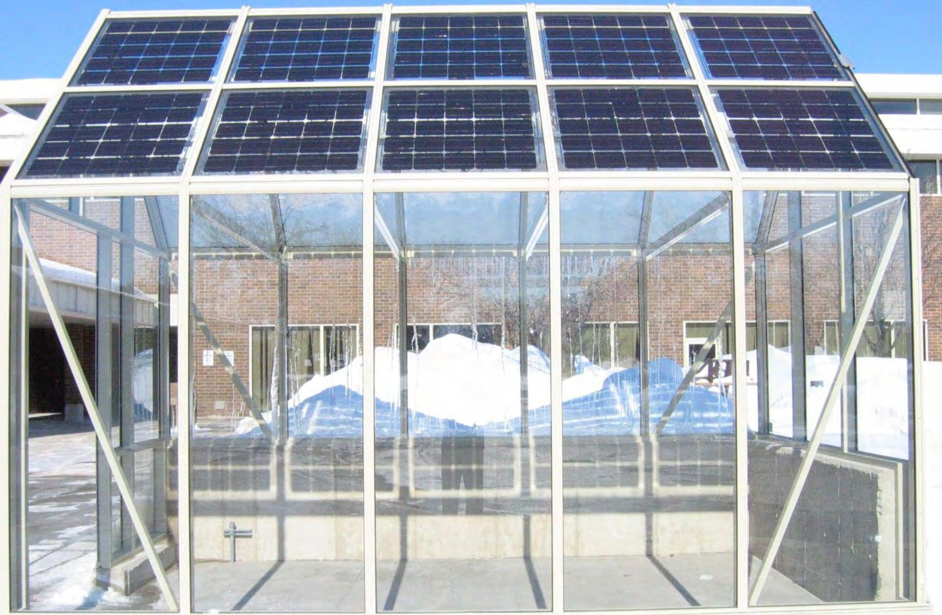
**Building Integrated Photovoltaic Bus Shelter – 1.0 kW (2007)**
